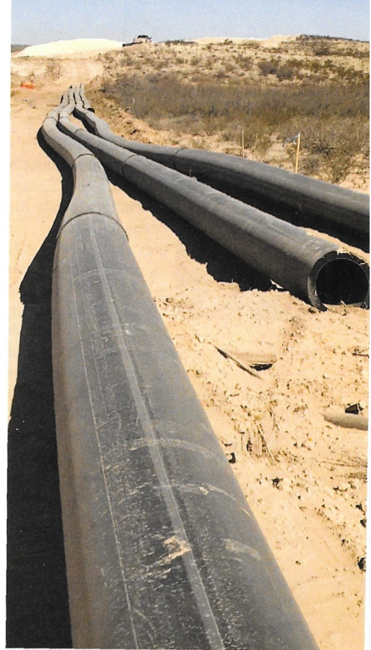
Some of the polyethylene pipe used in the project.
